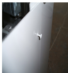
Fitting the lower panels
