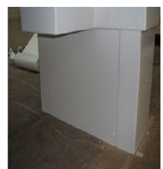
Securing the panels
